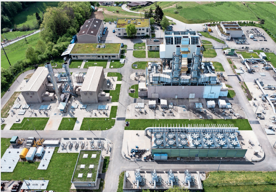
Fig. 3 Kompressorstation in Ruswil.
