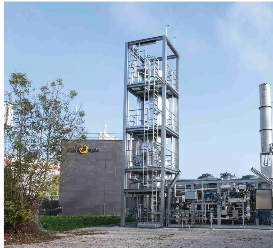
Hybridwerk Aarmatt © by Regio Energie Solothurn
